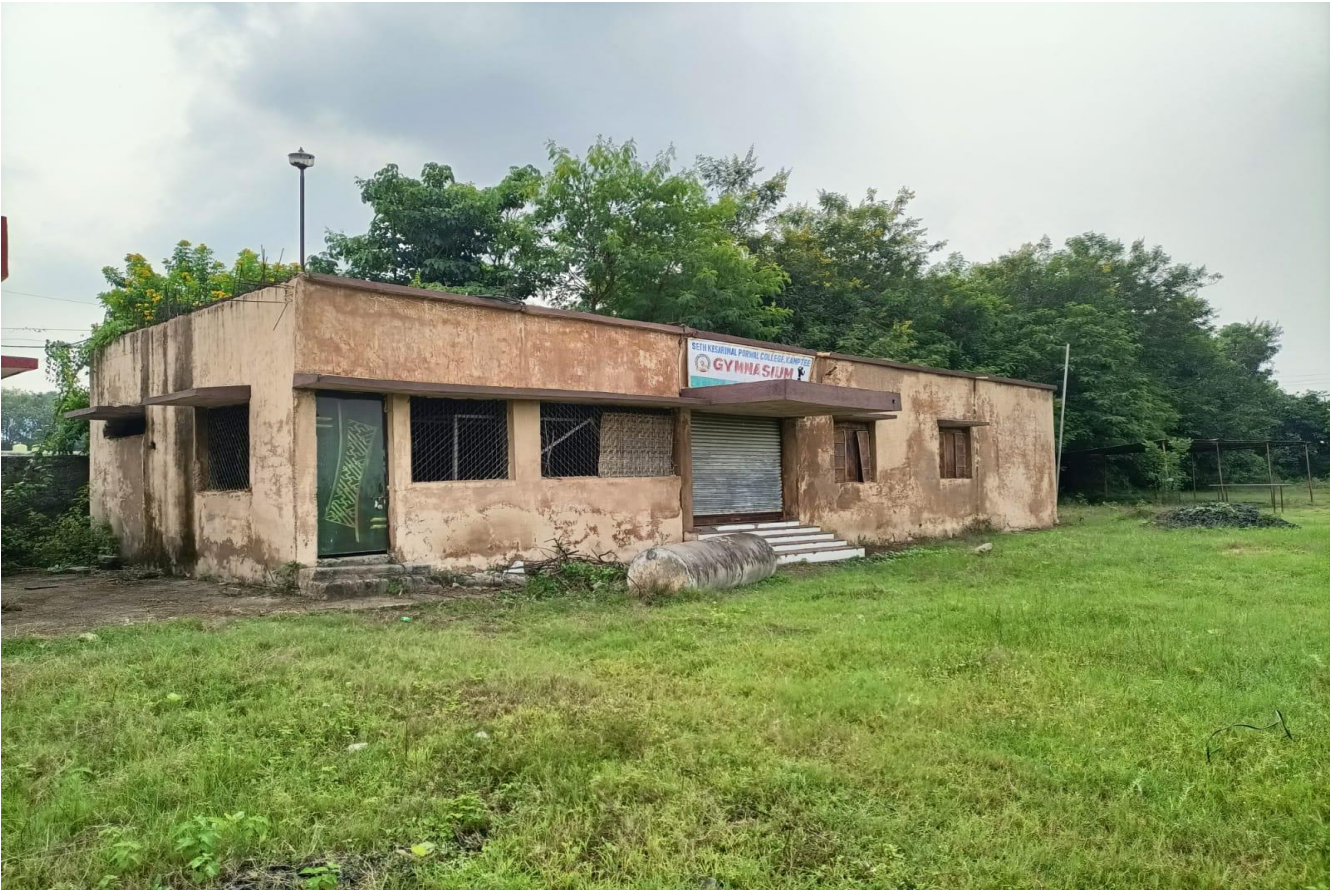
Multi Utility Hall
